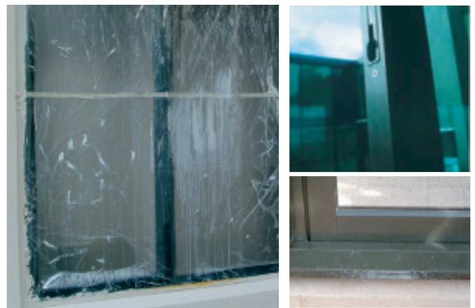
Three of these photographs display damage that has occurred on site, post installation. The photo of the masked joinery on the left displays clear signs of damage that could have occurred were it not masked. Please ensure that your joinery is protected right through the entire construction process.
